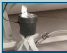
Installation of 120V. Pump
