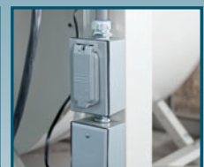
Provision & Installation of 120 V. Receptacles in SPC
