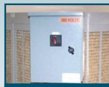
Installation of Weather proof NEMA 3R Box
