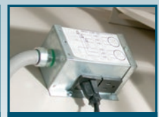
Installation of pump J-Box
