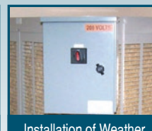
Installation of Weather proof NEMA 3R Box
