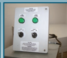
SPC switch box to control pump and fan operation
