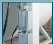
Provision & Installation of 120 V. Receptacles in SPC
