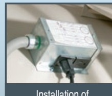
Installation of pump J-Box
