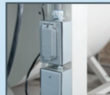
Provision & Installation of 115 V. Receptacles
