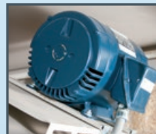
Installation of motor
