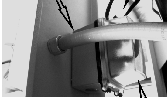
VISTA INTERIOR - PANEL CENTRAL
